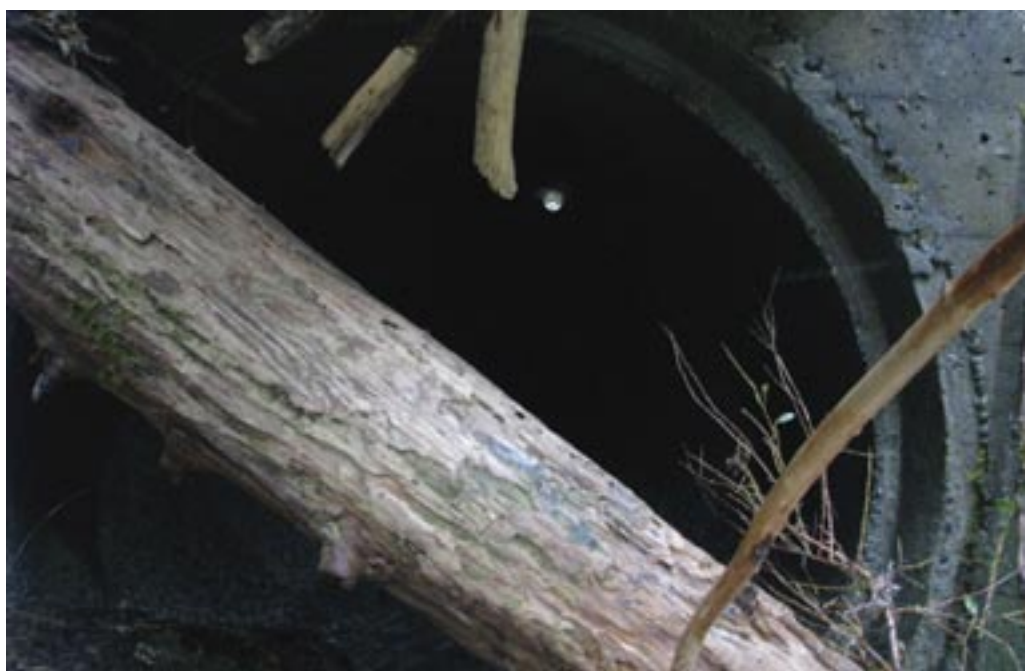
The culvert prior to reconstruction.
